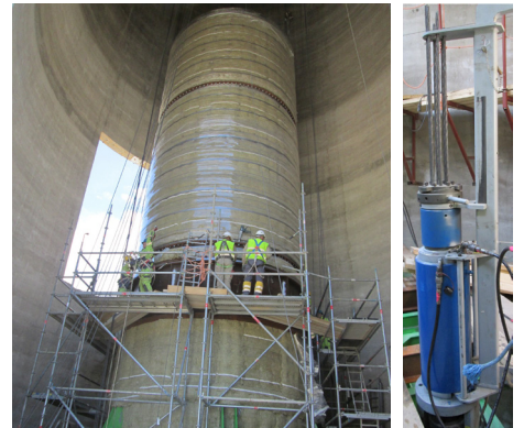
Inner liner assembly at the bottom of the stack. Heavy lifting jacks at the top of the stack
