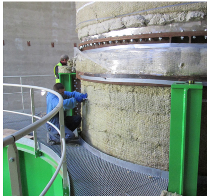
Liner fixed at the bearing platform
