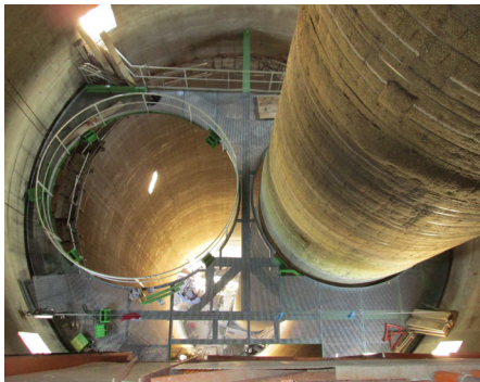
Liner fixed at the bearing platform
