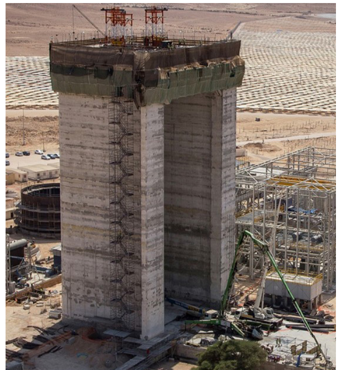
The north portion of the solar tower
